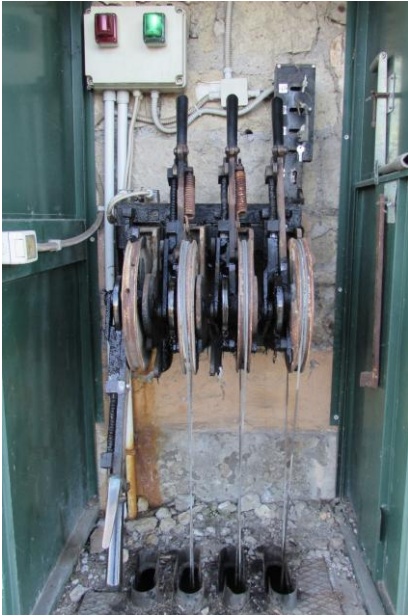
The interlocking system at Fabrica di Roma (photo taken by M.J. Santoni, 2019).
