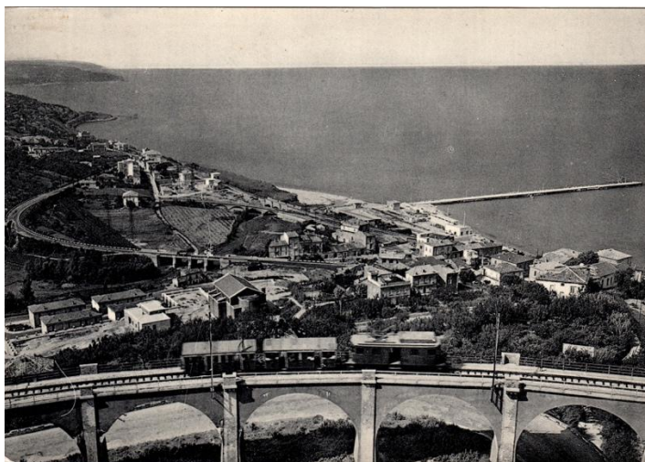
Rare image of the San Vito viaduct, when the line still was equipped with narrow gauge (unknown author, M.J. Santoni collection).
