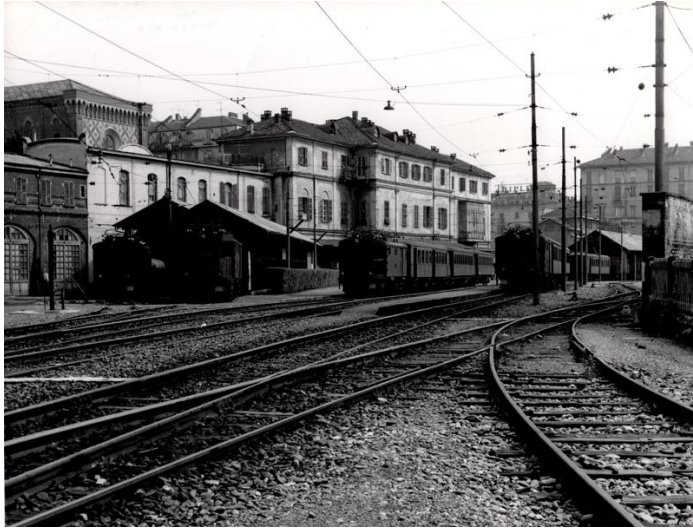
The railway yard of Torino Ponte Mosca station in the 1960s (photo taken by M. Boddi, M. J. Santoni collection).
