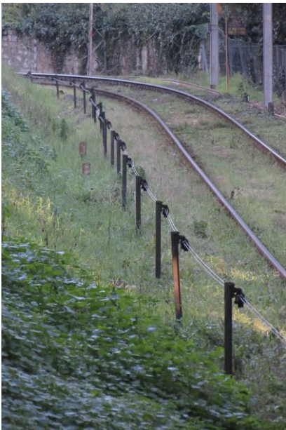
The double wire transmission that controls the semaphore in Vignanello station (photo taken by M.J. Santoni, 2024).
