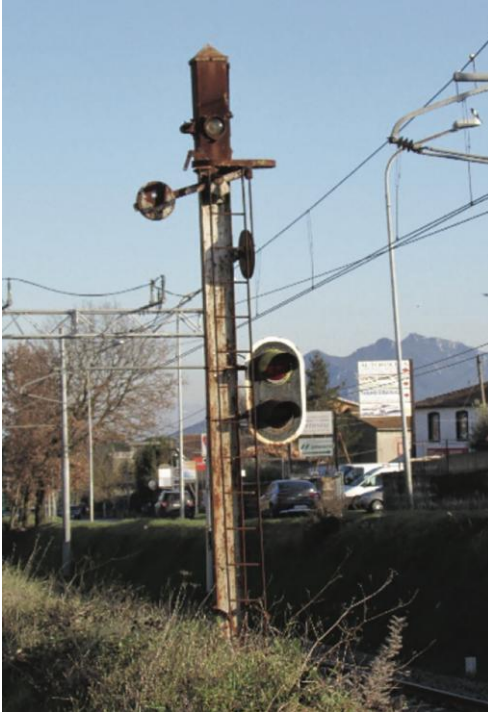
An example of how an element may be characterized by later additions and alterations. Depicted here is the Catalano station signal, originally of the mechanical type; the original structure was subsequently modified through the addition of electrical equipment and two signal lights. (photo taken by M. Boddi, M. J. Santoni collection).
