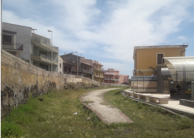
Abandoned Santa Maria di Licodia station, formerly part of the Circumetnea Railway surface alignment. Source: Giulio Pappa
