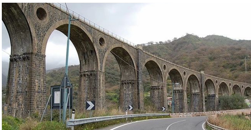
“S. Cataldo” Viaduct on the Alcantara-Randazzo line. Source: Sicilia in Progress
