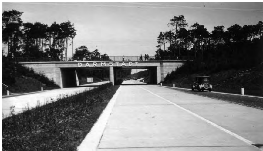
Figure 5. Autobahn at Darmstadt in 1936
